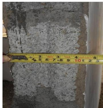
(g) The strength of the concrete used for construction had never been subjected to a laboratory test and instances where concrete not properly mixed and not up to the standard were observed in physical audit examinations. Eg- 25 Houses Project of lower part, 25 Houses Project- Henfold (Glen Eagles) part.
